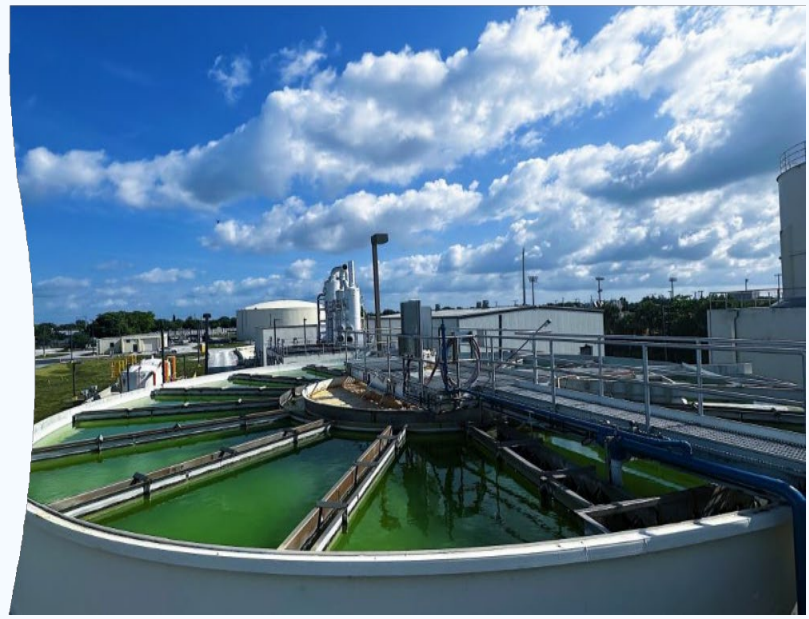
Picture 3: Lime softening accelerator
