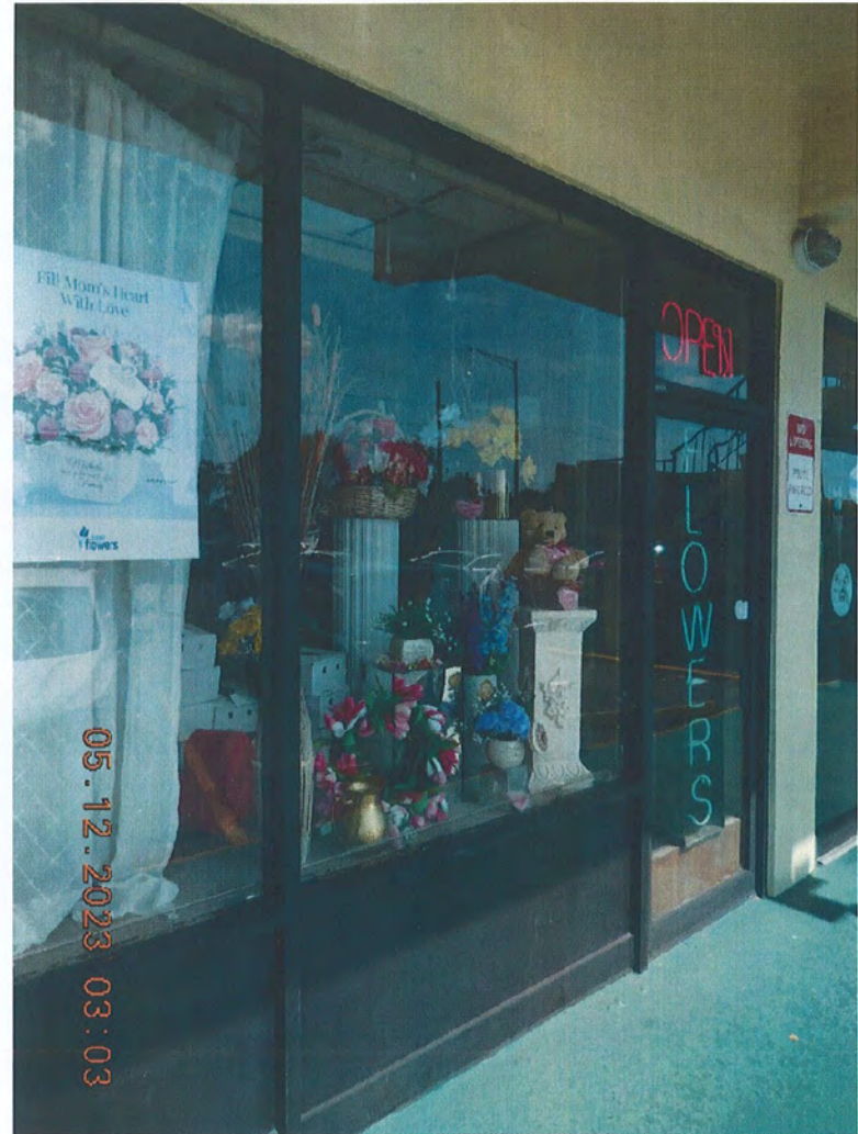
EXISTING STORE FRONT
