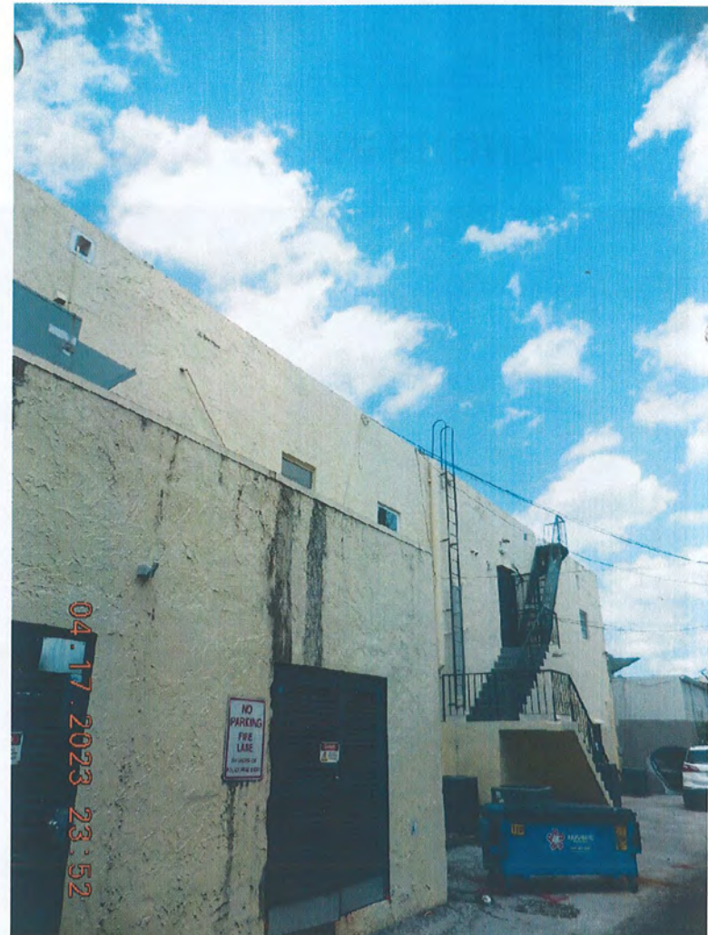
EXISTING NORTH END BACK OF BUILDING
