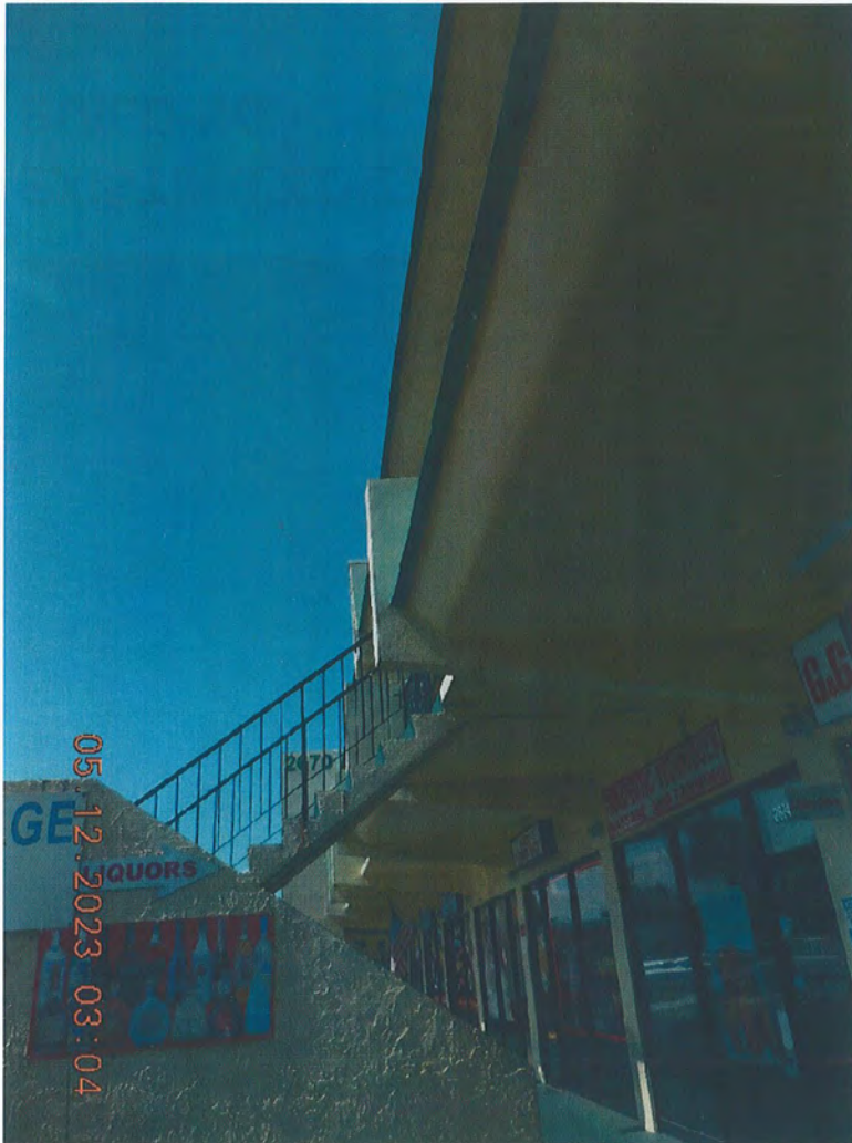
EXISTING GROUND FLOOR OVERHAND AND STAIR
