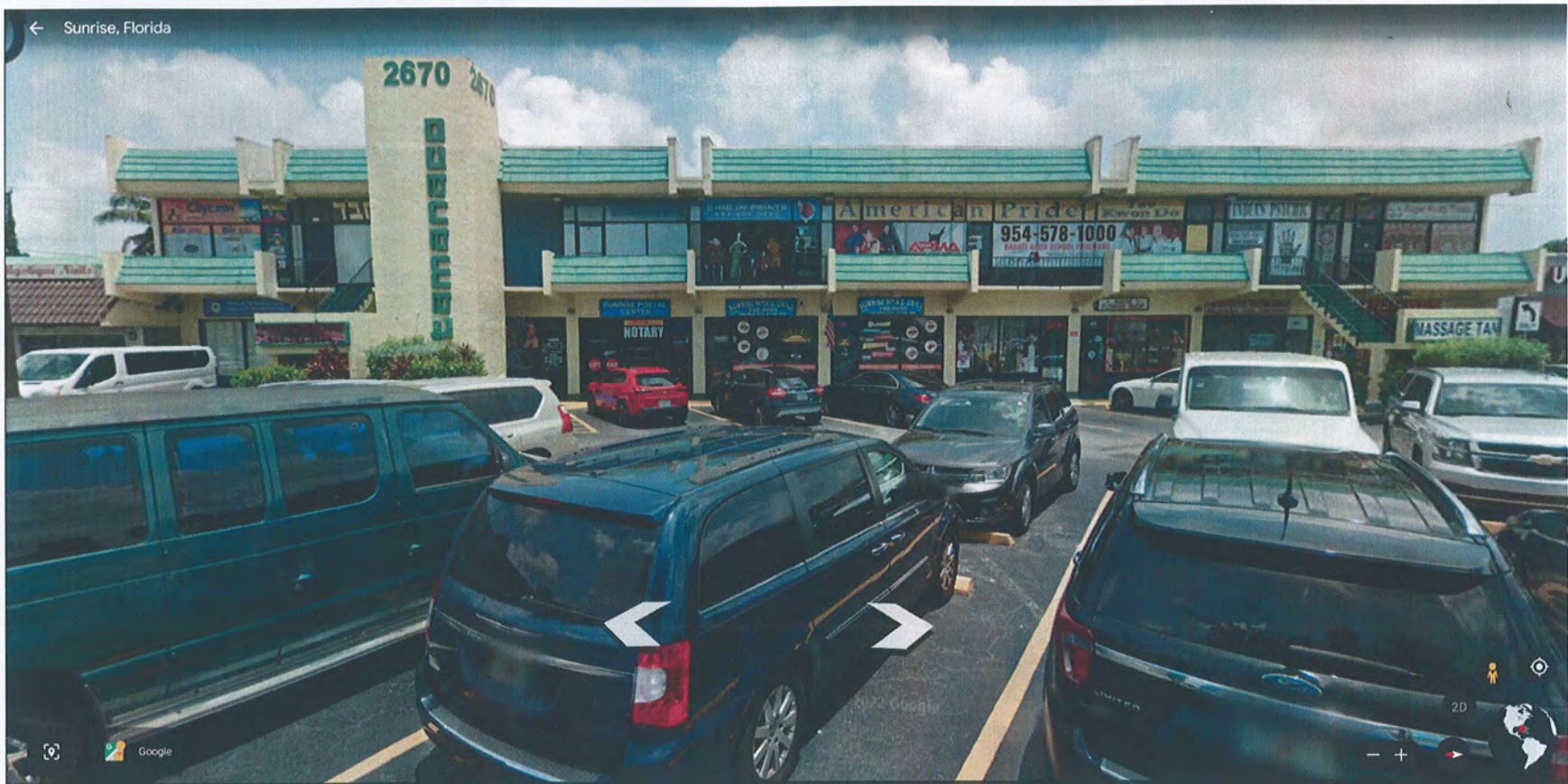
WEST FAÇADE OF EXISTING BUILDING
