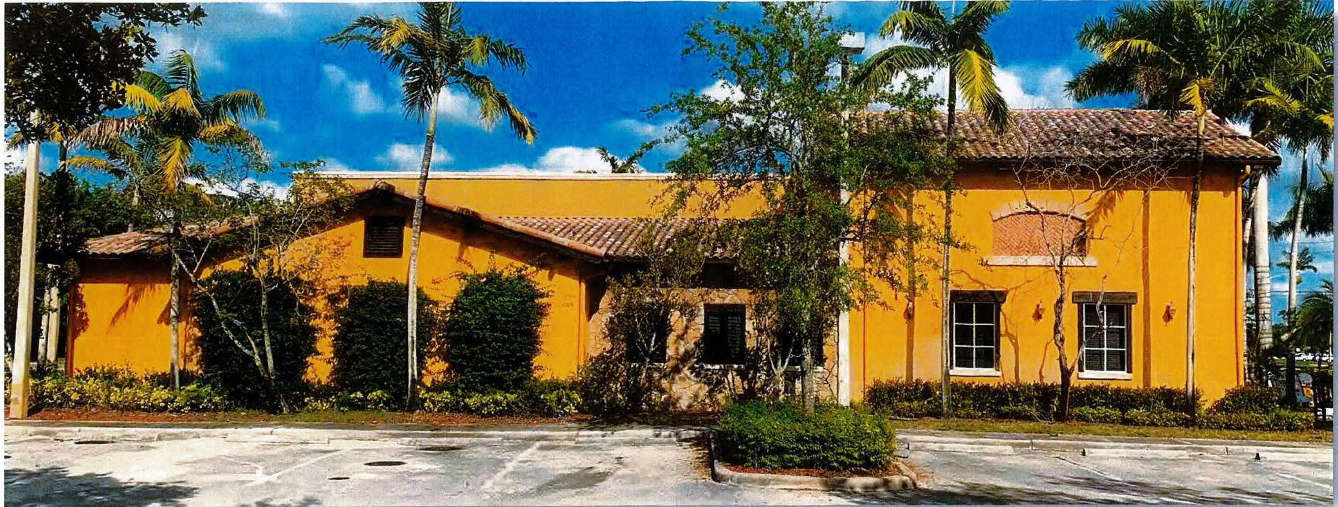
Image: West elevation of existing building. Photo taken from west parking area, facing east.
