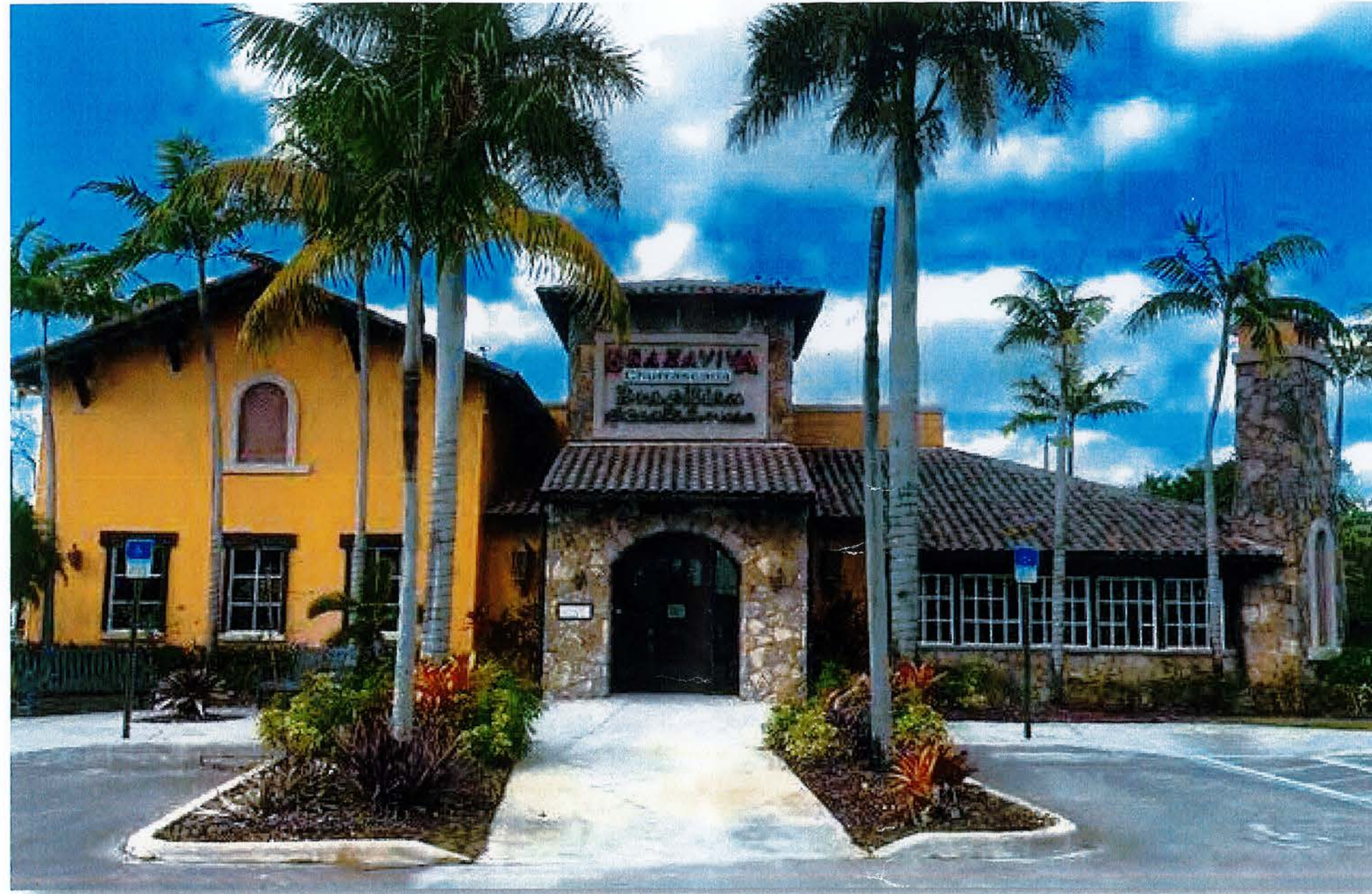
Image: South elevation, main entry facing Sunrise Blvd. Photo taken facing north.
