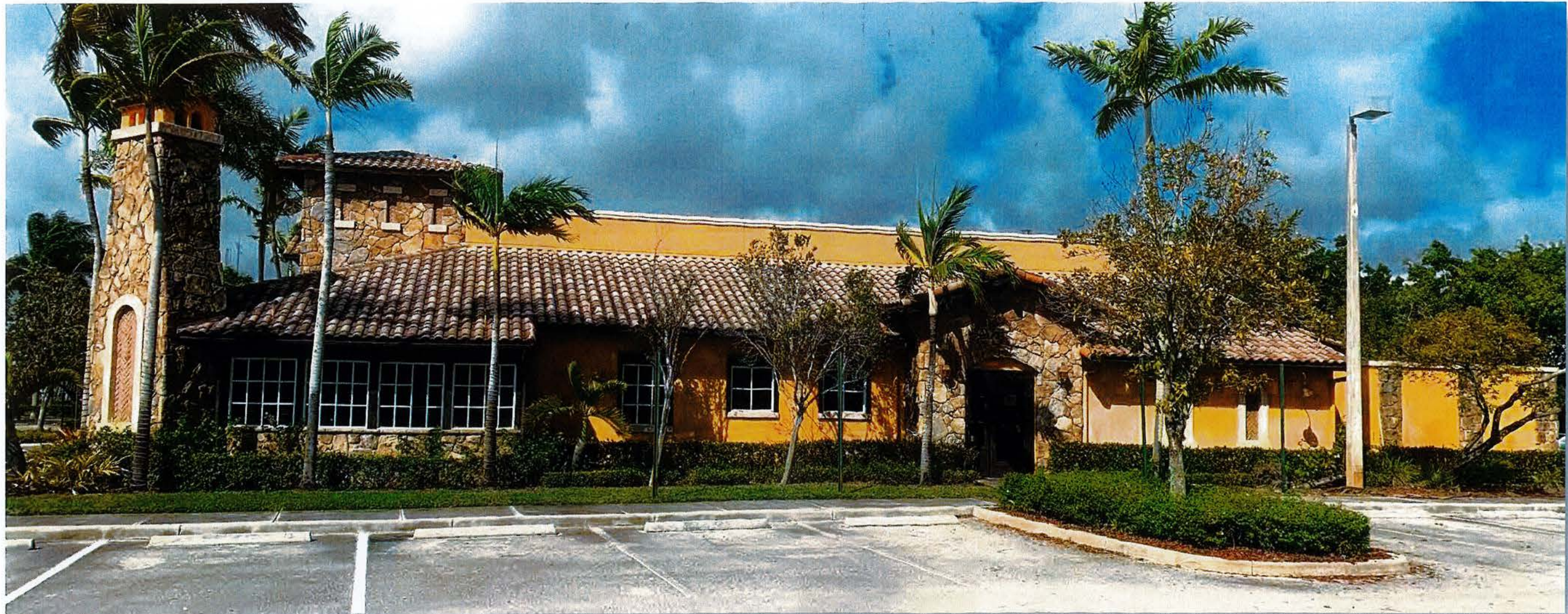
Image: East elevation of existing building. Photo taken from east parking area, facing west.
