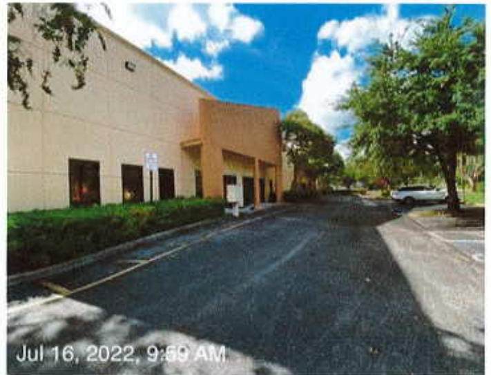
Front of Building-Building Facing West North Portion of Building
