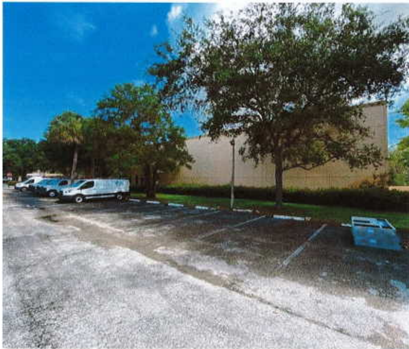
South Side of Building – Building Facing South
