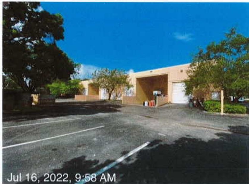
Rear of Building – Building Facing East
