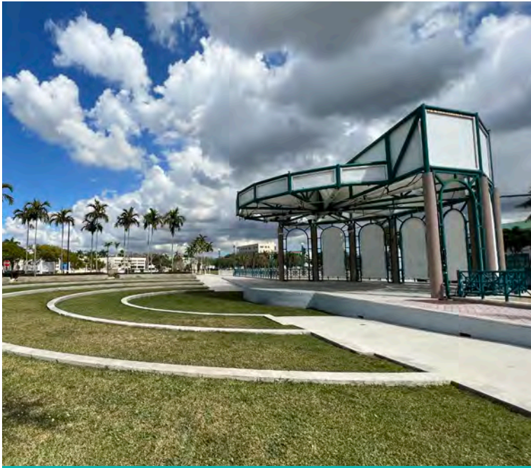
The Sunrise Civic Center Amphitheater is the home of the City's popular Tunes 'N Trucks concert series and other special events. An amphitheater expansion is planned as part of enhancements to the municipal complex.
