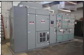
Unit Substation Transformer at Springtree WTP 500kva 4160volt - which provides power to the main switchgear in the Springtree WTP electrical room - requires replacement. This transformer was installed in the 1970's and has reached its useful life. Additionally this project will include the replacement of the Robicon Variable Frequency Drive (VFD) which operate the main high service pumps which have become obsolete and parts are difficult to obtain.
