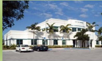
Gas Operations Building
