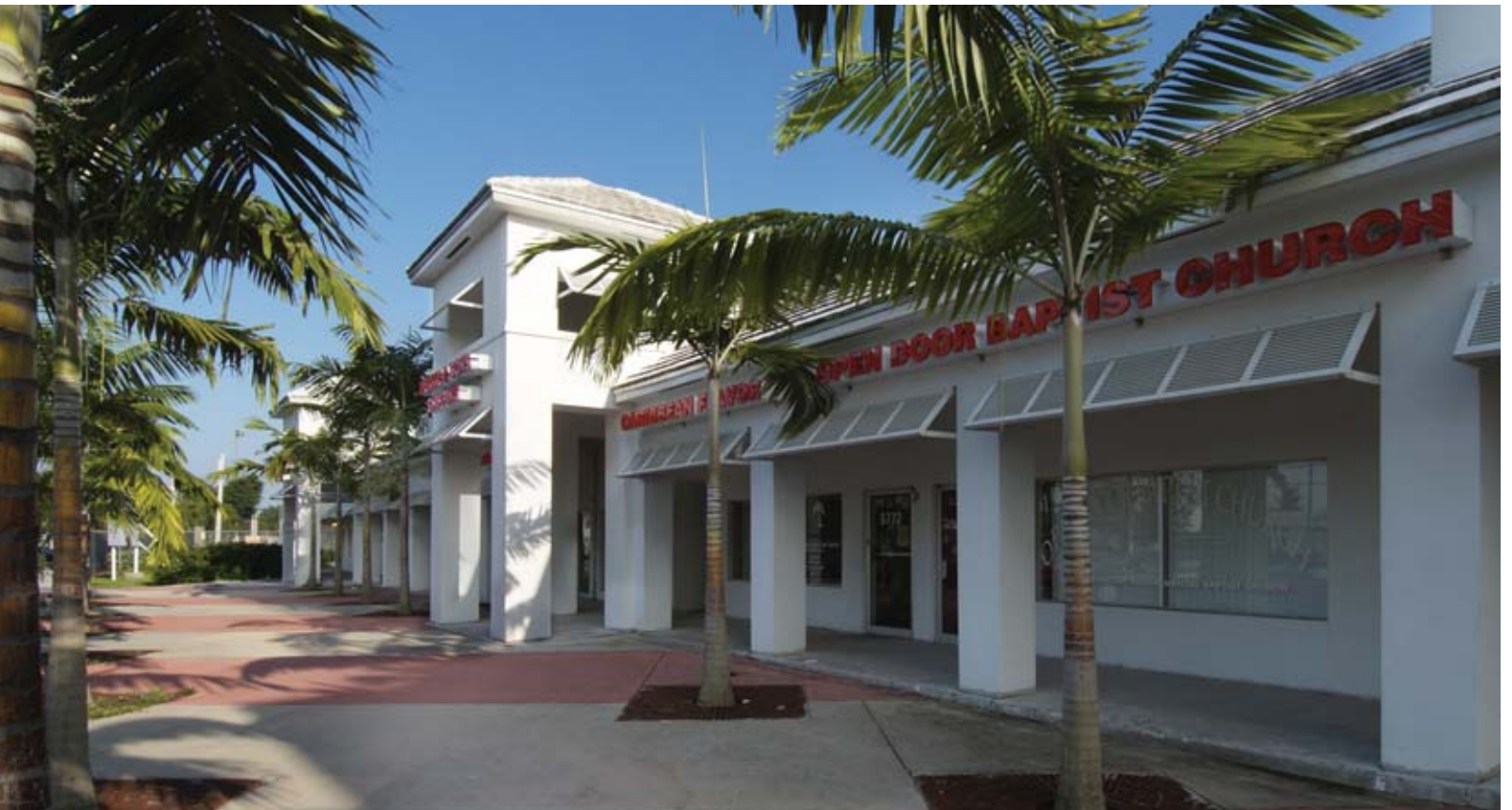
Phase II commercial façade enhancements, at the southeast corner of Sunset Strip and NW 68th Avenue
