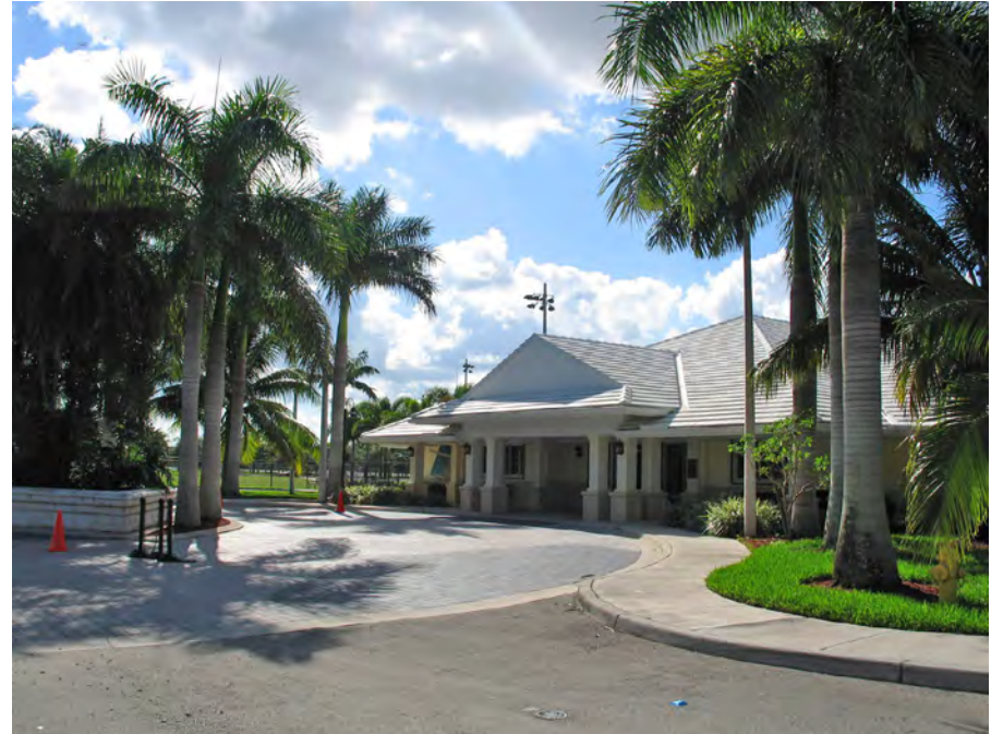
Meeting room at the New River Civic Center
